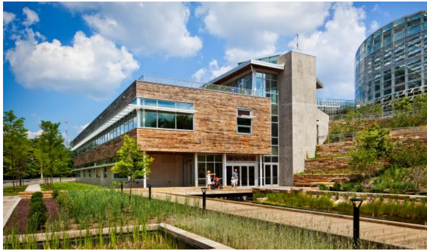
Figure 17. As-built view of the Center for Sustainable Landscapes (Schrag, 2017)
